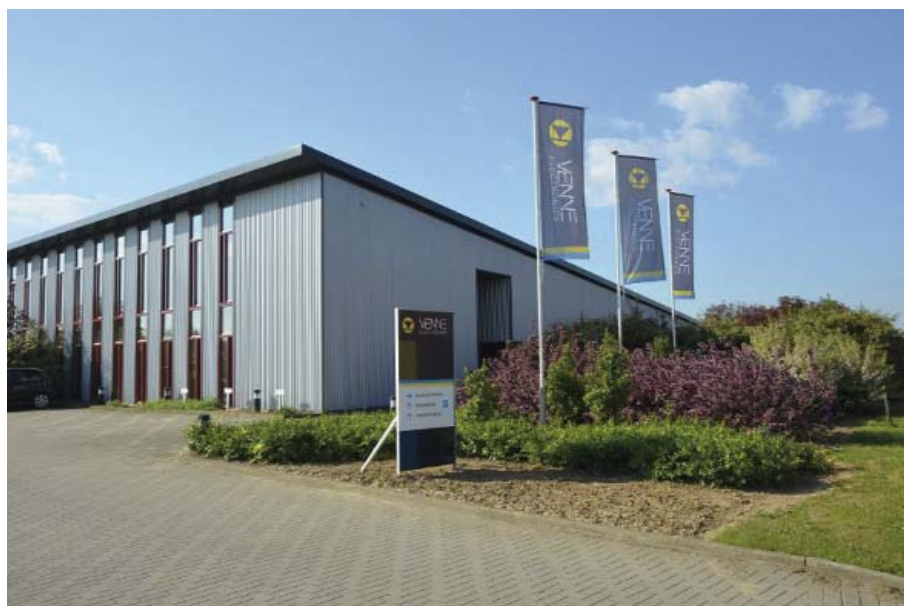
Das moderne Venne Electronics Headquarter in Maastricht in der Amerikalaan
